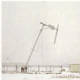
once the guy cables and the likewise pre-assembled electrical installation have been connected.
